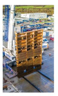
In conjunction with Scottish Canals and Eadon Design Consultants, AmcoGiffen managed this project from design to delivery, providing steel fabricated replacements of the upper and lower lock gate assemblies for Crinan Canal Locks 1 to 4, 14, 15 and Lock 17 at Gairlochy.
