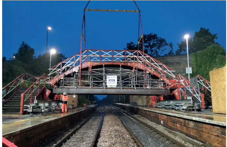
Removing the Existing Footbridge at Garforth Station
